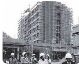
NWEC under construction (1976)
