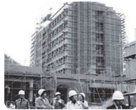
NWEC under construction (1976)
